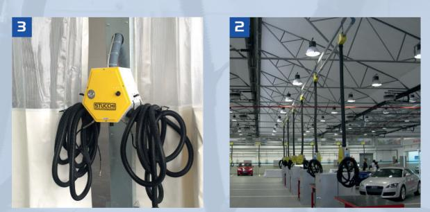
The EM model is suitable for a workstation, designed with a suction inlet in the lower part and with a manual device for the interception of the suction, air outlet and electrical socket dedicated for the connection to the Stucchi`s vacuum-cleaning central unit and allow the automatic start of the machine. It will be possible to activate the suction also trough the selector AUT/MAN (O/I) installed on the cover.
